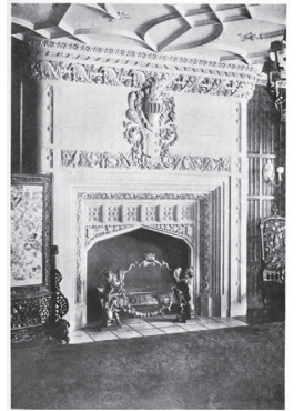
One of the many fireplaces at Longwood. Before demolition, architectural fixtures and relics from the home were salvaged or sold at a public sale.
