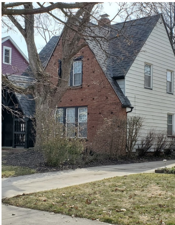
A home in Cleveland Heights sporting a T-Lock Shingle roof.
