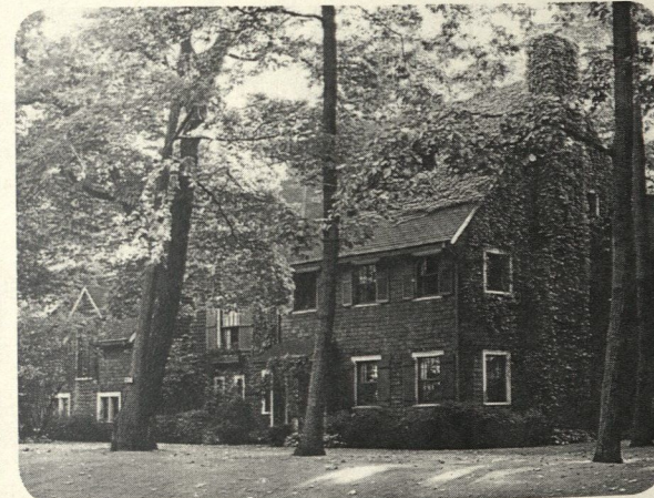
11936 Carlton Rd. Demolished.
