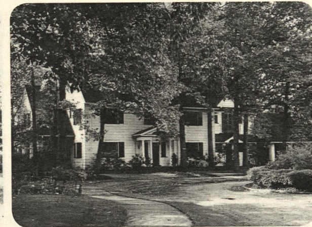
11896 Carlton Rd. Demolished.
