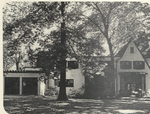
11930 Carlton Rd. Demolished.
