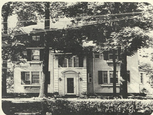
11905 Carlton Rd. Demolished.
