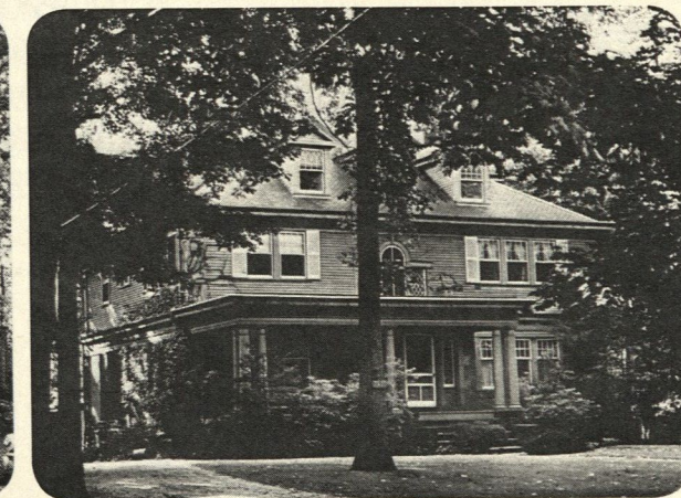
11900 Carlton Rd. Demolished.
