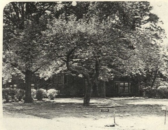
11894 Carlton Rd. Demolished.
