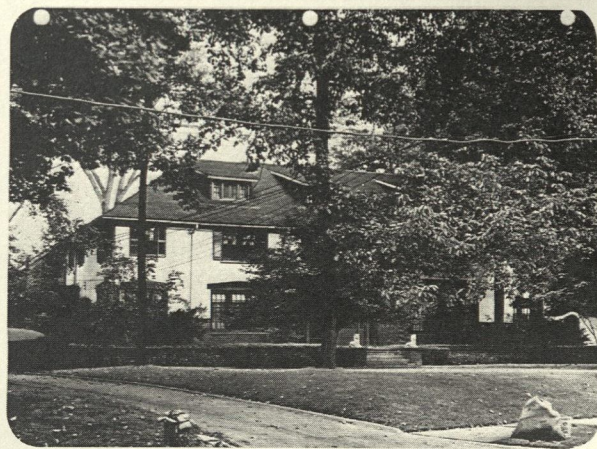
11945 Carlton Rd. Demolished.
