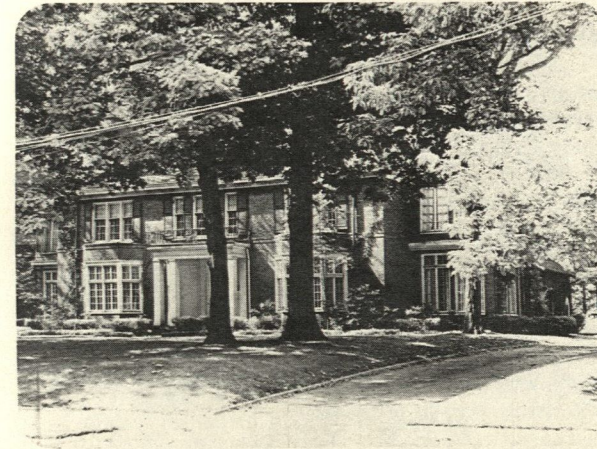
11931 Carlton Rd. Demolished.
