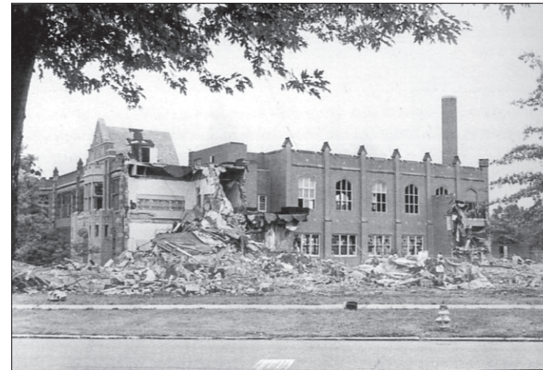
Figure 13. Taylor School demolition.
