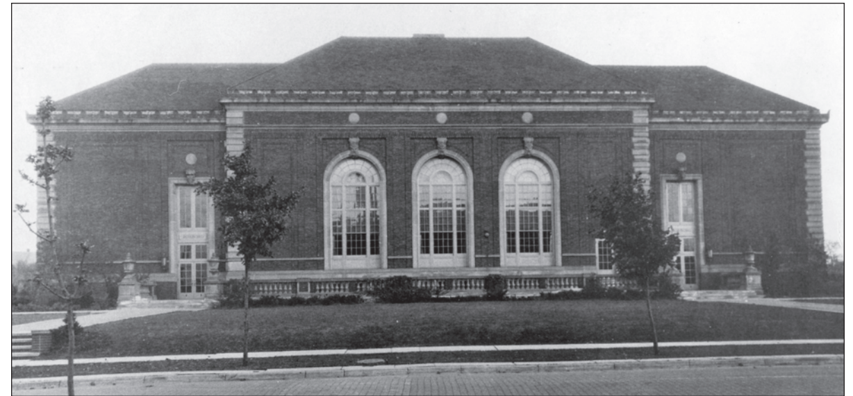
Figure 7. The "new" Roxboro Elementary.
