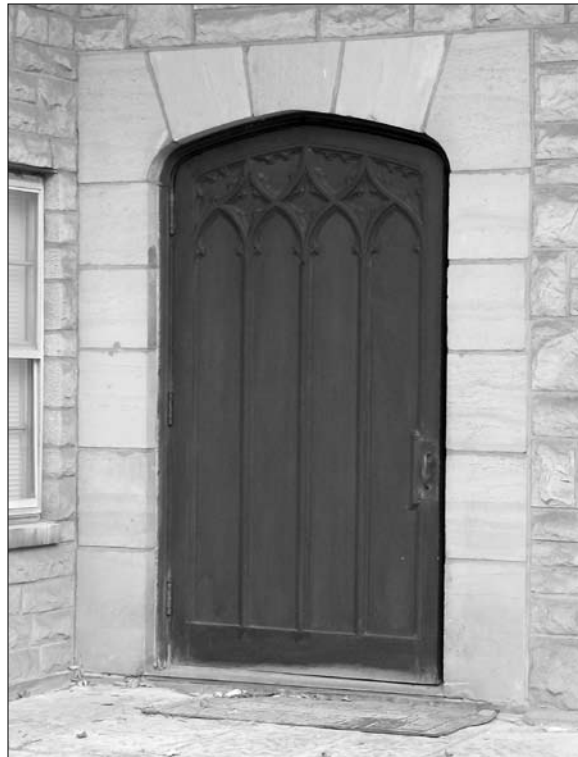
Figure 2: The developers of Overlook Park Apartments incorporated the front door of the old Eels mansion into their design.
